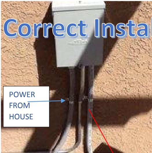
Install 50 Amp Breaker in main panel box in house. Run wires from breaker out to where the spa is going and install subpanel as per instructions in pre-delivery guide.
